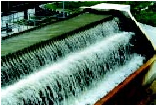
Loji pembersihan air di Wangsa Maju, Kuala Lumpur. Water treatment plant at Wangsa Maju, Kuala Lumpur.
