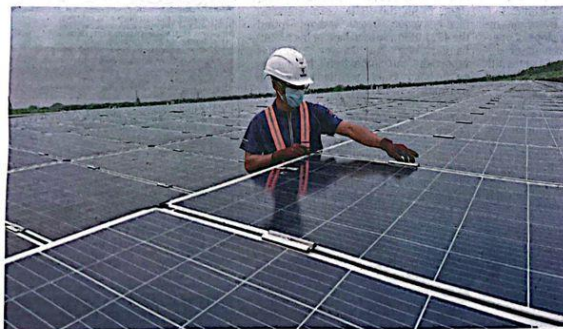
Green initiative: The third-party access concept will continue in the form of Corporate Green Power Programme where participants can produce and sell renewable energy to their off-takers via the grid.
