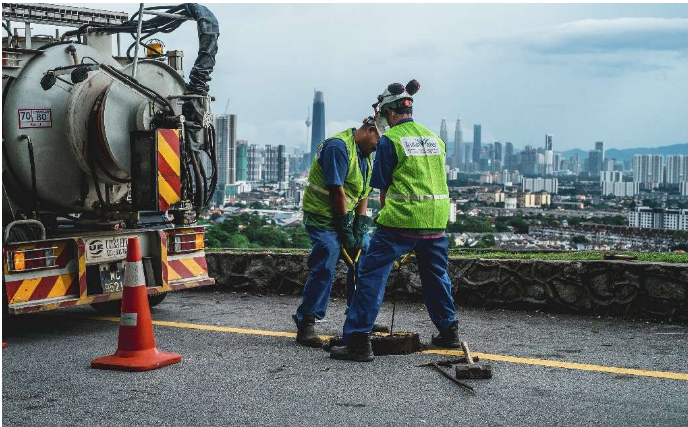
IWK team performing sewer network maintenance
